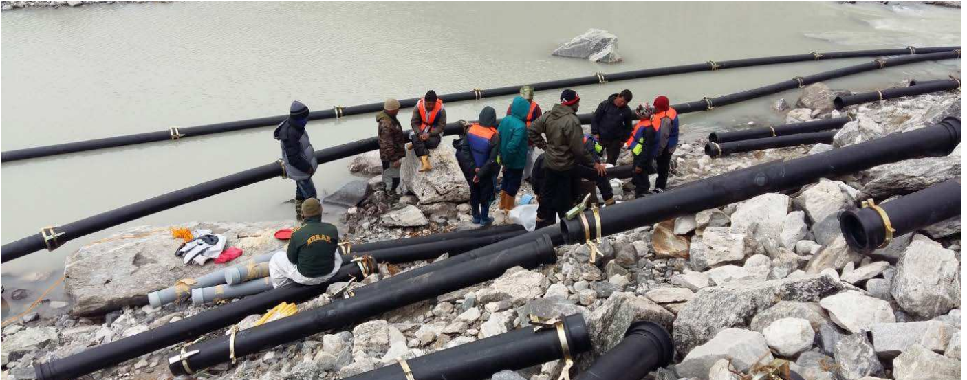
Installation of siphon system
